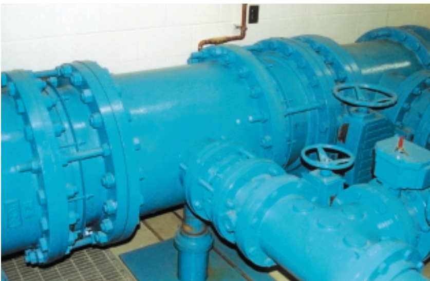
Crown WTP, Cleveland, Ohio, US
